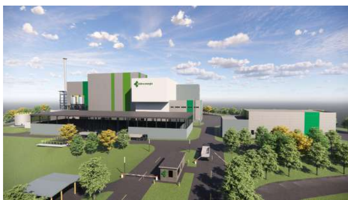
Figure 2. Visualisation of the new WtE plant in Olsztyn, Poland, which will thermally treat 110 000 tpy of refuse-derived fuel from the region when completed.
