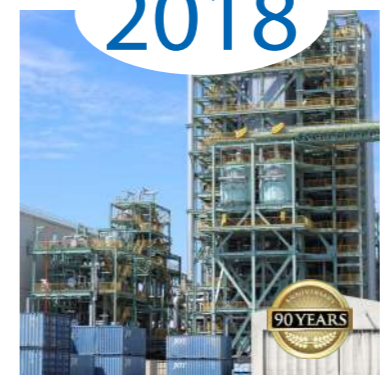
90 th company anniversary Supply of CFB technology for the first fully biomass-fired power plant in Japan
