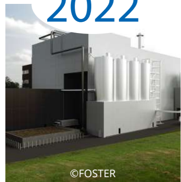
Successful re-entry into the market for thermal sewage sludge treatment by winning the contract to supply the new Flanders plant in Belgium
