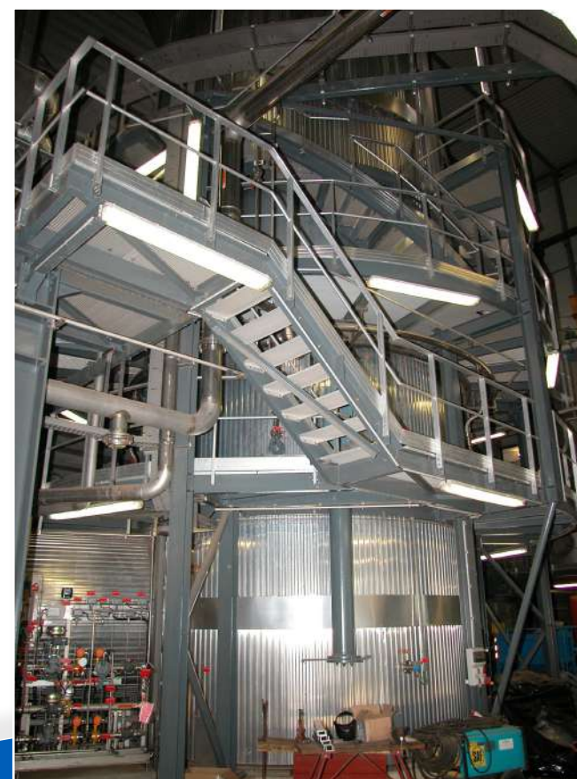
Stationary fluidised bed furnace for the incineration of municipal sewage sludge (sewage sludge incineration plant, Pierre Benite, France)
