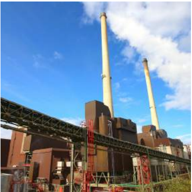
Moneypoint, Ireland 3 x 305 MW e Circoclean® flue gas cleaning system
